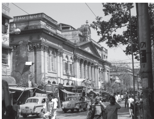
Fig. 3: Clockhouse of Mullick on Chitpur Road.
