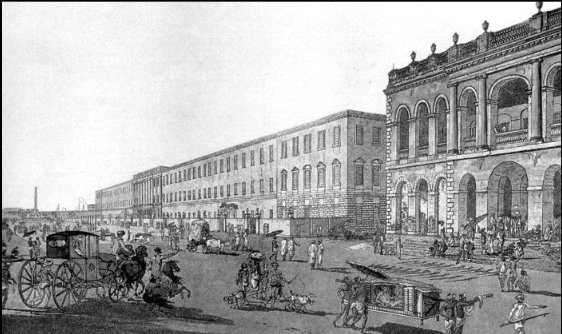
WRITERS' BUILDING Built in 1780 Designed by : THOMAS LYON
